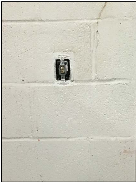
Photograph 6. Missing Switch Plate in Automotive Shop
